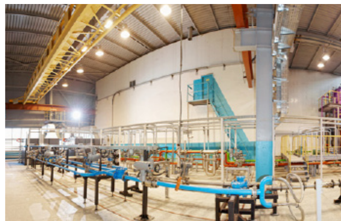
Multiphase metrological test flow facility
